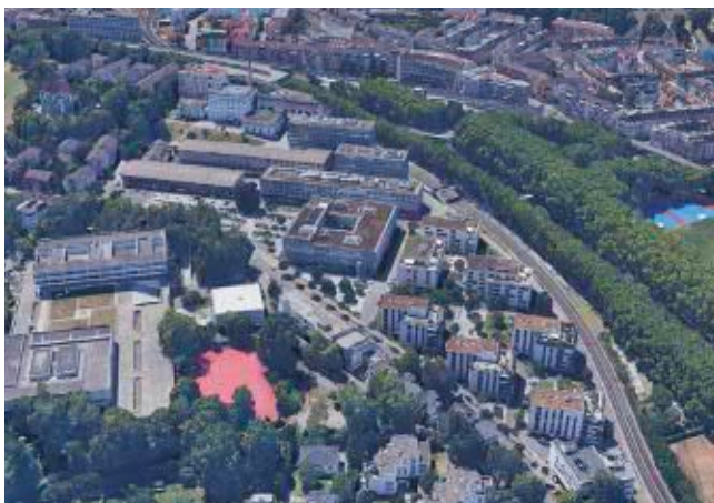
Abb. 3 Hürliemann-Areal (Google Earth)
